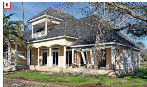
Figure 5. Comparison of residential structures in Port St. Joe elevated above BFE (a) and built at grade (b). (From (FEMA, 2020))
