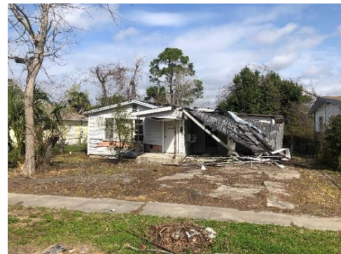
Figure 4. Example of wind damage caused by Hurricane Michael in North Port St. Joe; roof cover damage (left) and roof cover damage and structural collapse (right)
