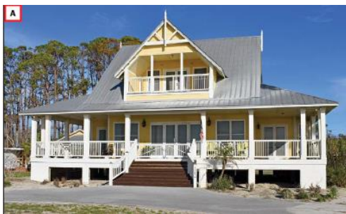
Figure 5. Comparison of residential structures in Port St. Joe elevated above BFE (a) and built at grade (b). (From (FEMA, 2020))
