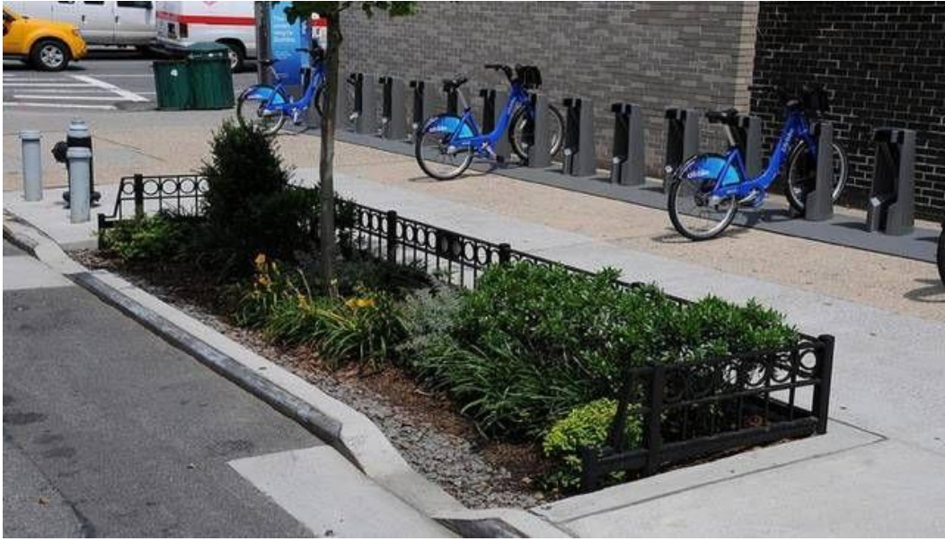
Figure 13 Example of a biowale in sections
