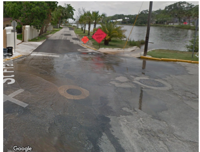
Figure 3. Nuisance flooding at the intersection of Cordova and St. Francis Streets.
